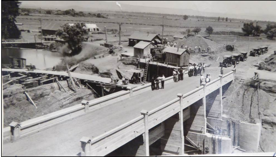
Figure 3: Pit 1 Gatehouse 9-10-11 under construction, circa 1922. Fort Crook Museum Photograph Archive, Fall River Mills.
