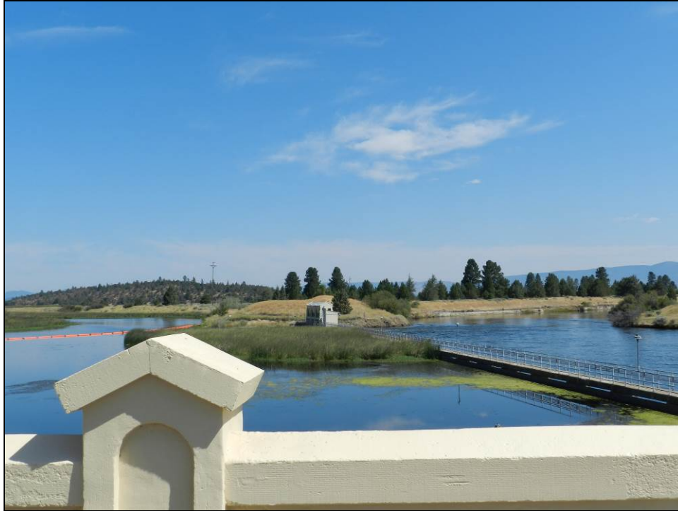
Figure 48: View of Gatehouse 1-2-3 from the roof / former road deck of Gatehouse 9-10-11. Camera facing north, August 16, 2016.
