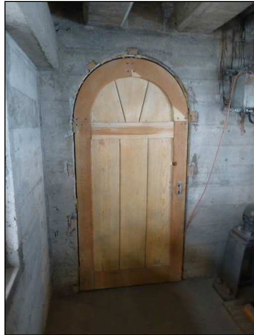
Figure 33: Original door on west side of Gatehouse 9-10-11, stripped, May 19, 2016.
