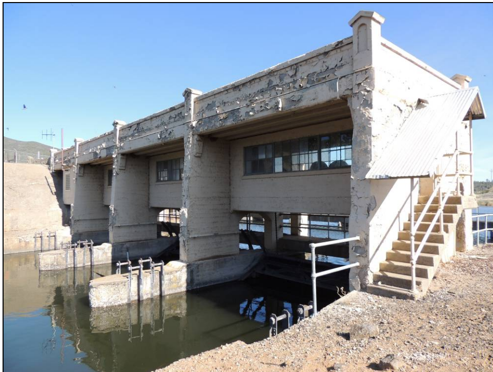
Figure 9: Pit 1 Gatehouse 9-10-11, April 2014. Note concrete spalling along exterior of former bridge deck.
