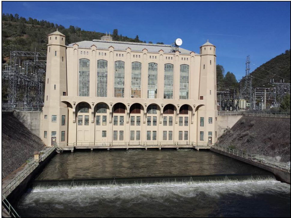
Figure 2: Pit 1 Powerhouse. Other components of the Pit 1 Hydroelectric System are architecturally unified around this highly stylized Gothic Revival edifice.
