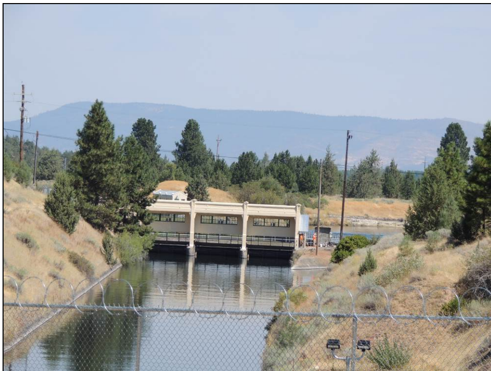
Figure 47: Gatehouse 9-10-11 as seen from Glenburn Road, August 16, 2016.
