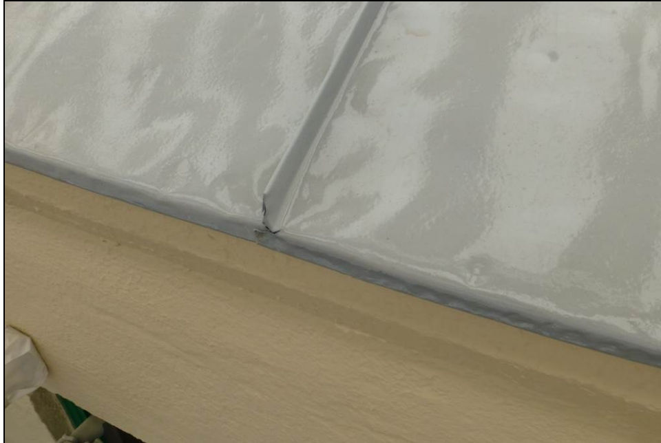
Figure 36: Detail of a coated raised-seam tin roof, Gatehouse 1-2-3, January 27, 2016.
