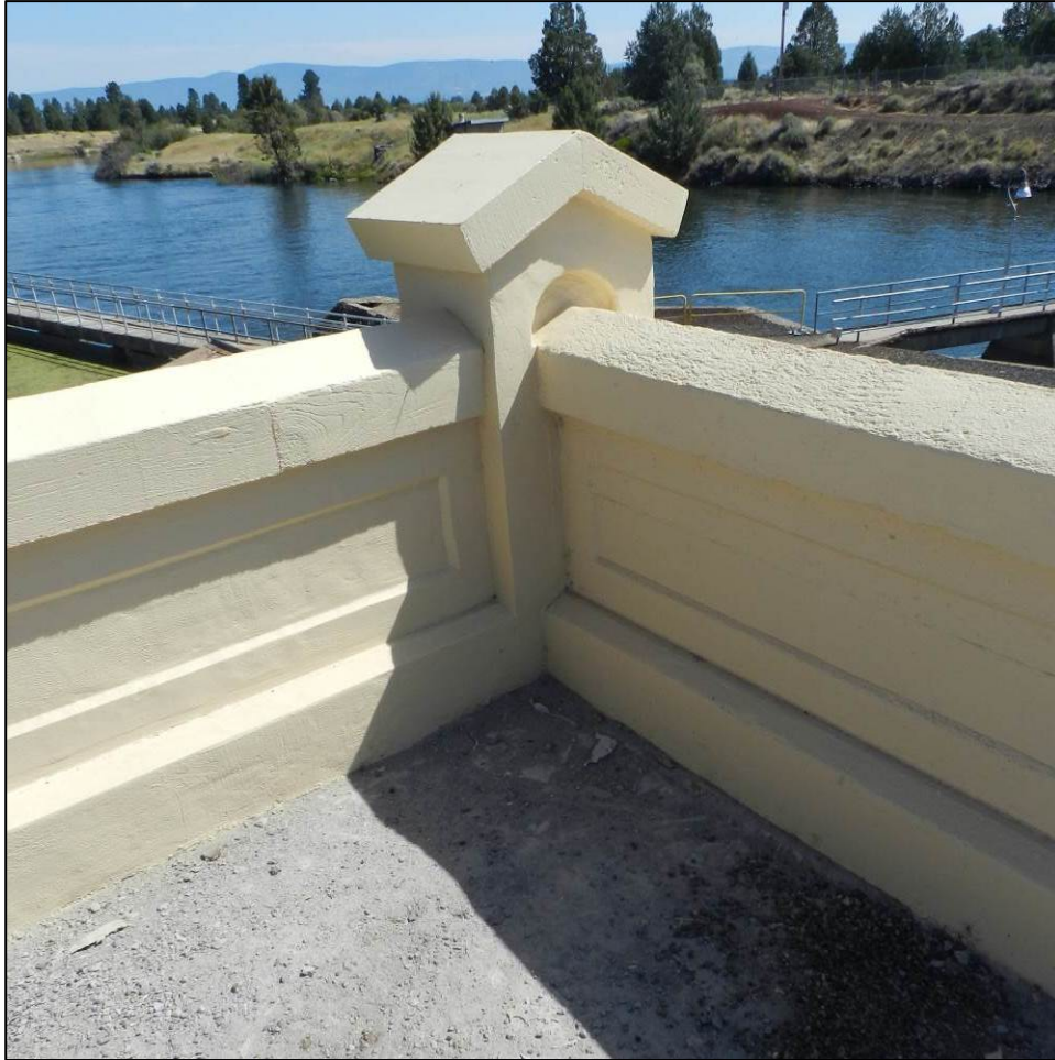
Figure 44: Detail of reconstructed architectural detail at northeast corner of Gatehouse 9-10-11, August 16, 2016.
