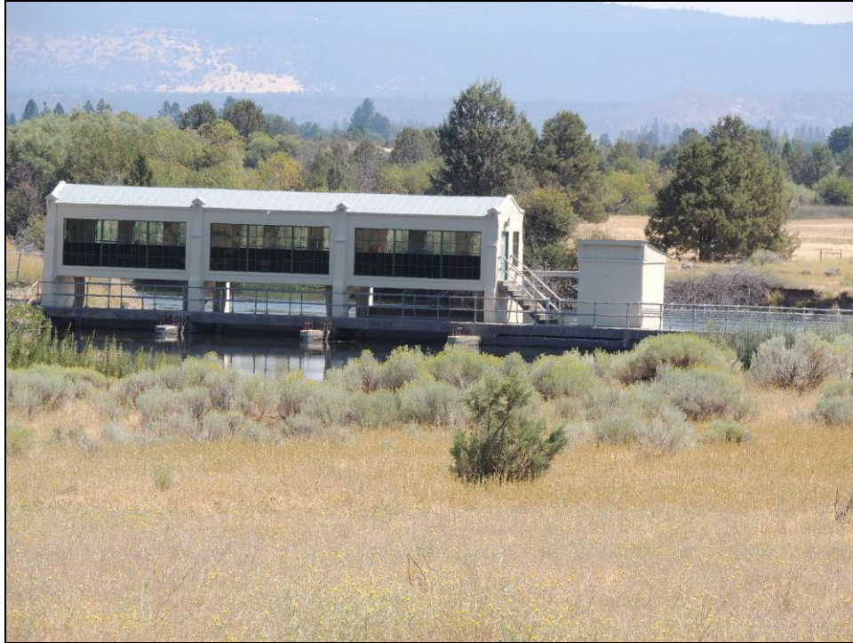
Figure 46: Gatehouse 1-2-3 as seen from Glenburn Road, August 16, 2016.
