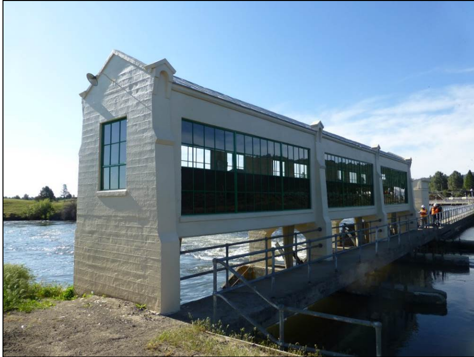
Figure 28: Pit 1 Gatehouse 1-2-3, May 19, 2016. Note that laminated glass windows provide security while allowing visibility through building. Also note reflection of light off rows with black film at far right.
