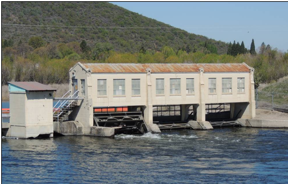
Figure 14: Pit 1 Gatehouse 1-2-3 at right and Float House at left, April 2014. Note roof addition on Float House and replaced window panes on gatehouse.
